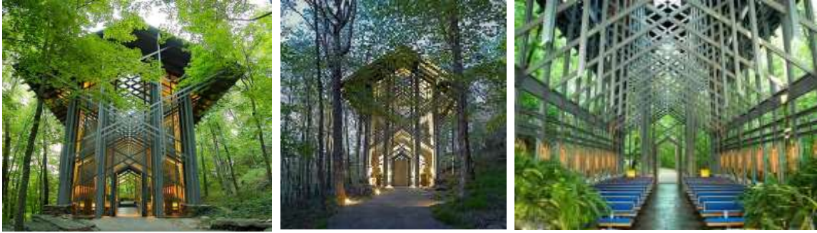
Figure9. Thorncrown Chapel Structure, designed by Euine Fay Jones
